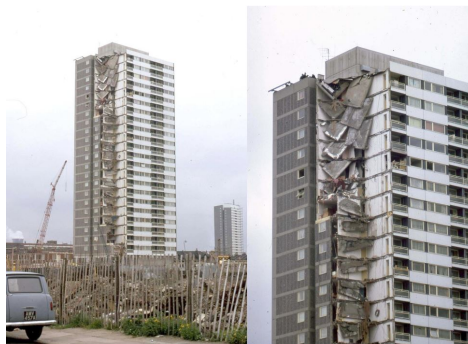
FIG. 6. Ronan Point Tower crash on May 16, 1968, in East London (photo: Derek Voller, Ronan Point collapse, Canning Town, CC BY-SA).
