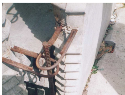
FIG. 9. Vertical connection of wall panels [26].
