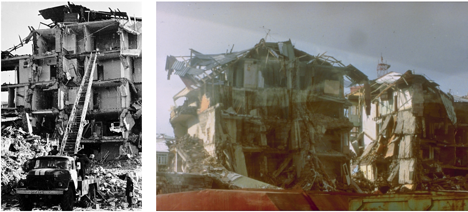
FIG. 7. Damage caused by the 1988 earthquake of Spitak (Armenia) (authors of photos: Vsatinet, CC BY-SA 4.0 (on the left); C.J. Langer. U.S. Geological Survey, public domain (on the right)).
