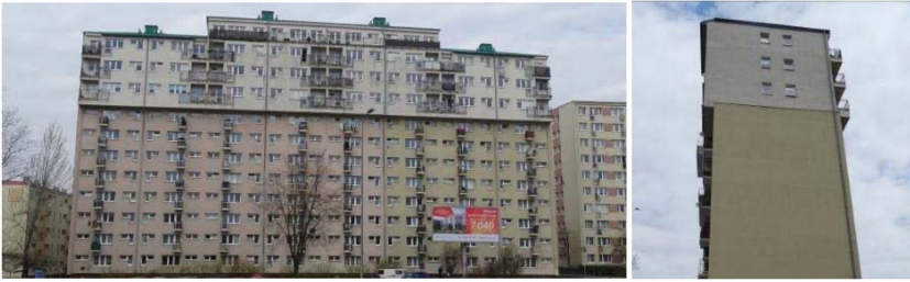
FIG. 1. The superstructure on an existing LPS building (photo: P. Knyziak, CC BY) [13].
